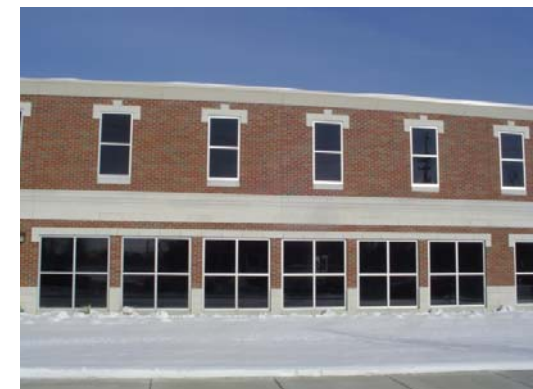
Side facing faux windows, which break up a long building facade
