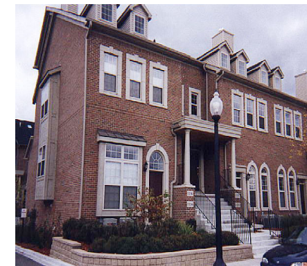
Building facades should include the use of compatible materials, colors and textures.
