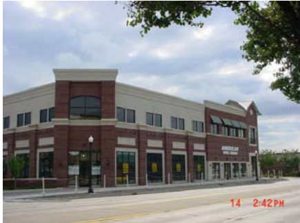
The long façade is broken up by several storefront bays.
