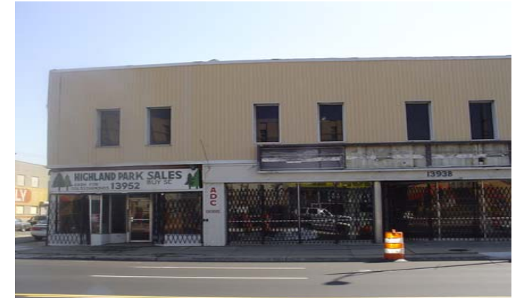
Security gates such as these should not be permitted. All gates should be located behind the window displays so the view into the building and the goods offered are fully visible.
