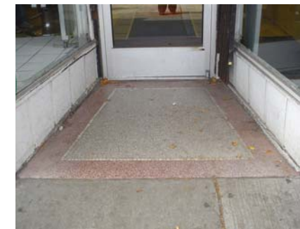
Interesting details like this terrazzo paving entry to the storefront can be installed as it adds distinctive character to the area.
