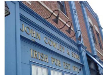
Wall signage (applied letters) should be visible without overwhelming the building face or extending over the sill of the second floor level, as seen in this example.
