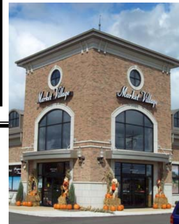
Corner Business Sign
